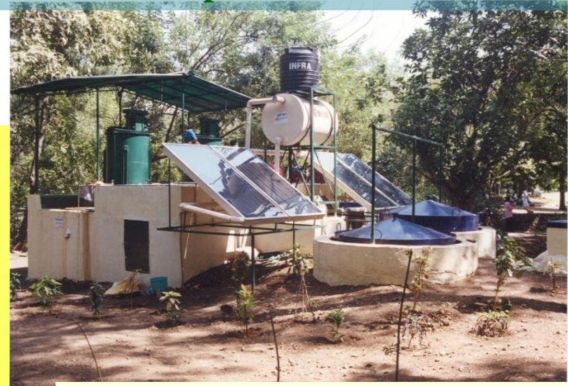
NISARGRUNA Plant for disposal of Biodegradable wastes
